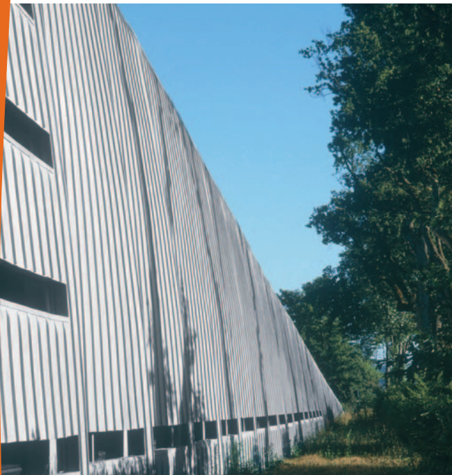
Noiseproof wall in VM ZINC ® Blanquefort (France) Architect(s): Déesse 23
