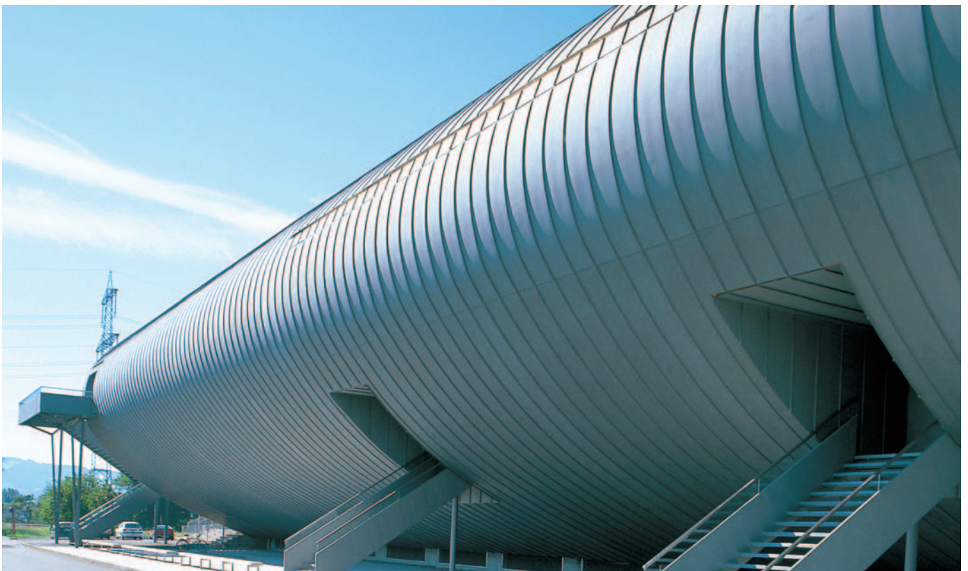
Multi purpose hall, Dornbirn (Austria) Architect(s): Kaufmann 96 GmbH Contractor(s): Fa. ERO, Fa. Helmut Rümmele
