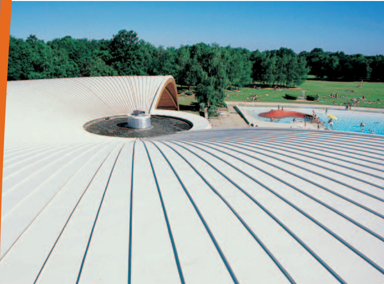
Swimming pool, St Quentin en Yvelines (France) Architect(s): Carduner
