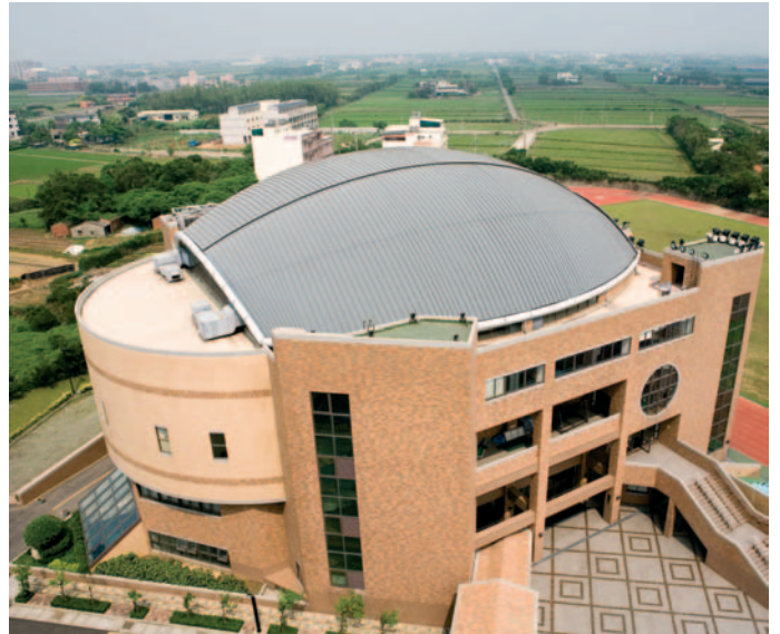
China Technical College, Hsinzue (Taiwan) Architect(s): Tien-Hao Huang Architecture & Associates Contractor(s): Bluescope Lysaght Taiwan
