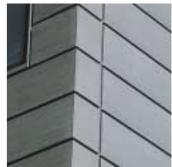
The strips are profiled in the workshop and are attached by interlocking with a grooved lip to give a recessed joint effect. They are attached to the wood or metal framework by hidden fixing clips on the inside edge of the grooved lip.
