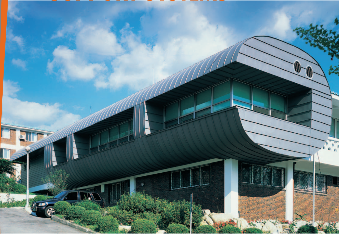
Kangwon University - Dormitory, Chuncheon (South Korea) - Architect(s): San - Contractor(s): Sunnie International
